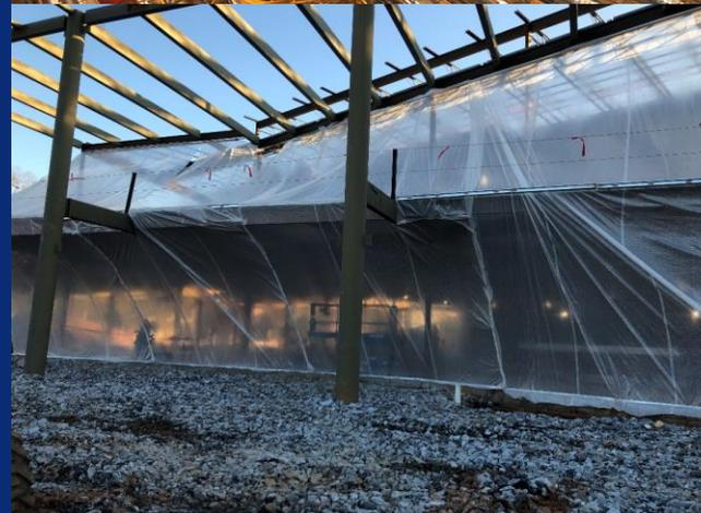
Main and 2<sup>nd</sup> level provided with temp heat and enclosure to facilitate 2<sup>nd</sup> level concrete pour
